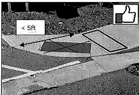
Solution 1. DWS may be located at the bottom of the ramp when located less than 5 ft from back of curb.
