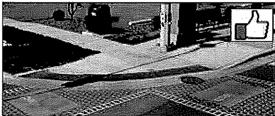
Detectable Warning Surface is the full width of the ramp.
